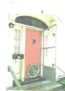
Blower-door testing provides a
