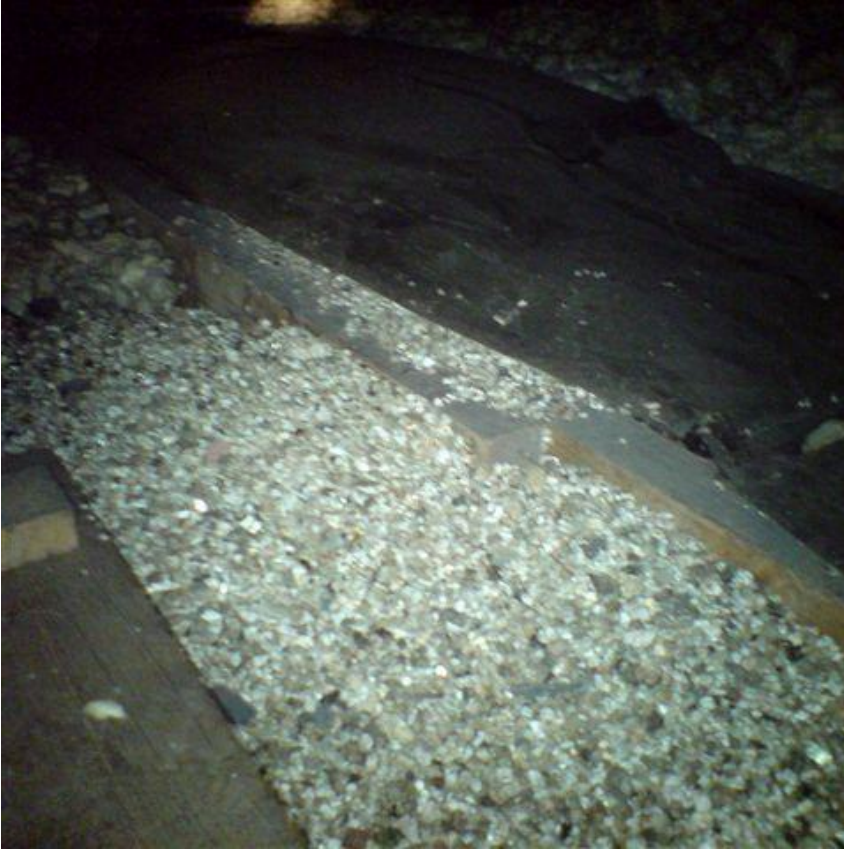
Vermiculite insulation with asbestos
