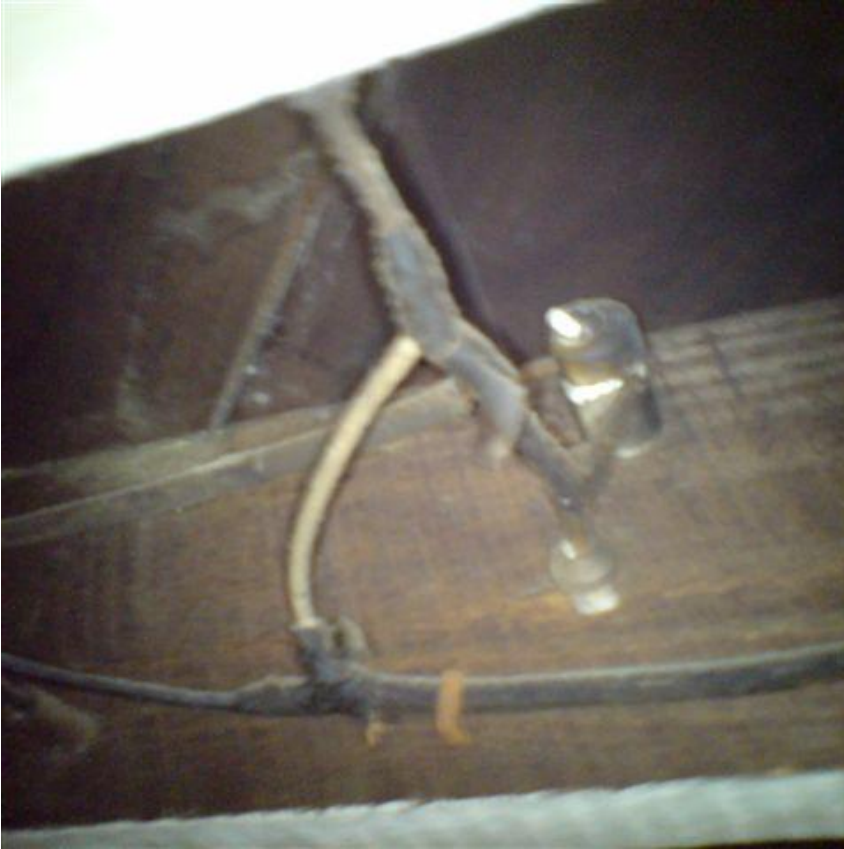
Unprotected Knob and Tube wiring connections not inside of a junction box
