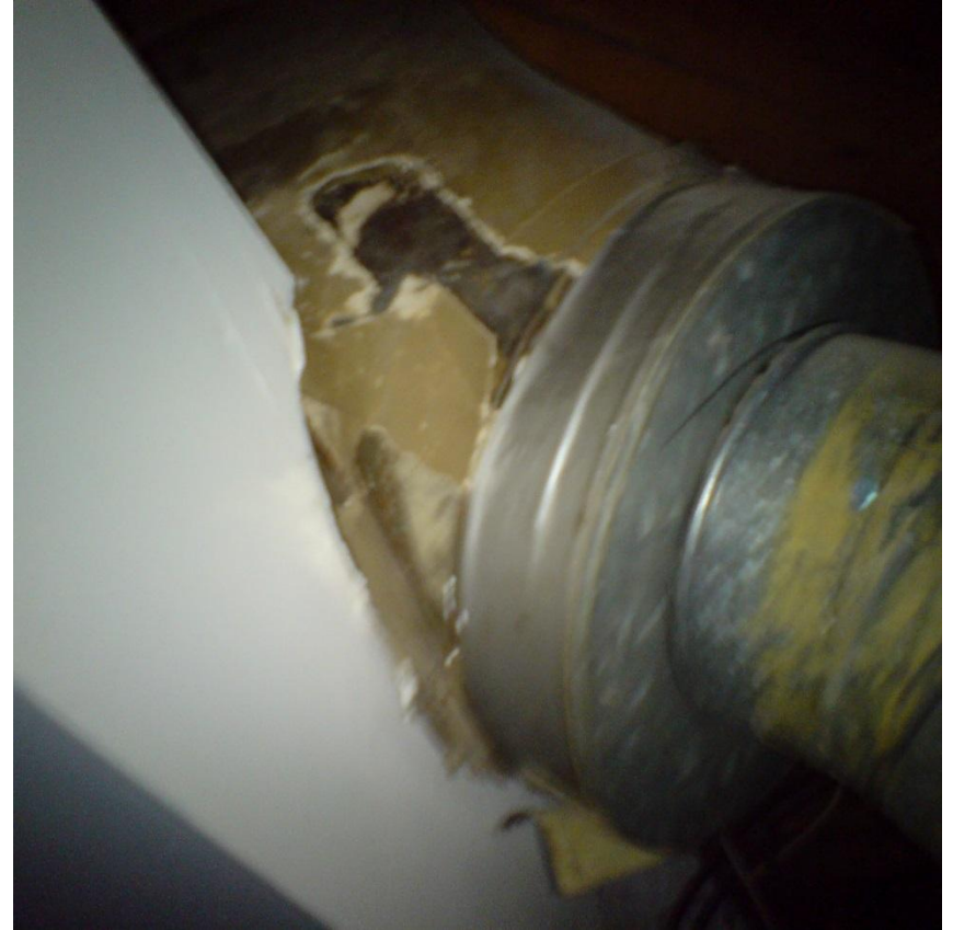
Friable asbestos around duct
